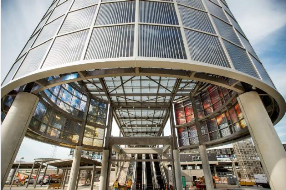
BART Warm Springs / South Fremont Station
